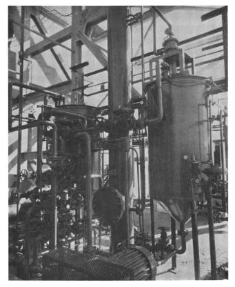
Figure 4. Ion exchange softening
